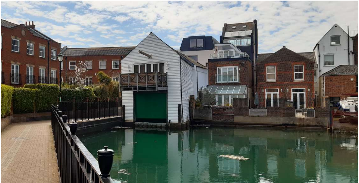
Rear (north-east) of site, in white-painted weatherboard timber cladding, facing the Inner Camber.
